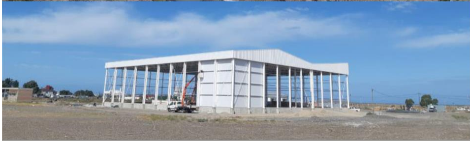
Construction Work New IQF Shrimp Production Line. Rawson
